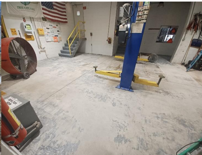
SHOP FLOOR PREP
